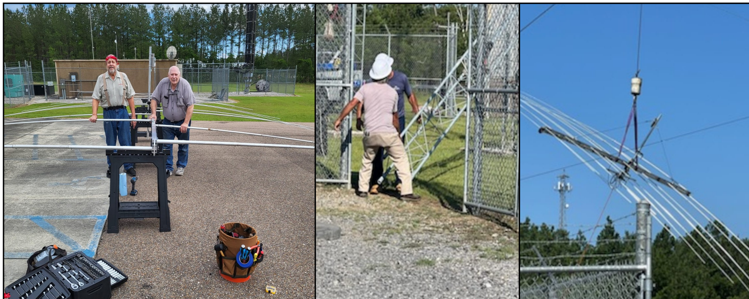
Progress photos on new tower erection for Washington Parish EOC location
